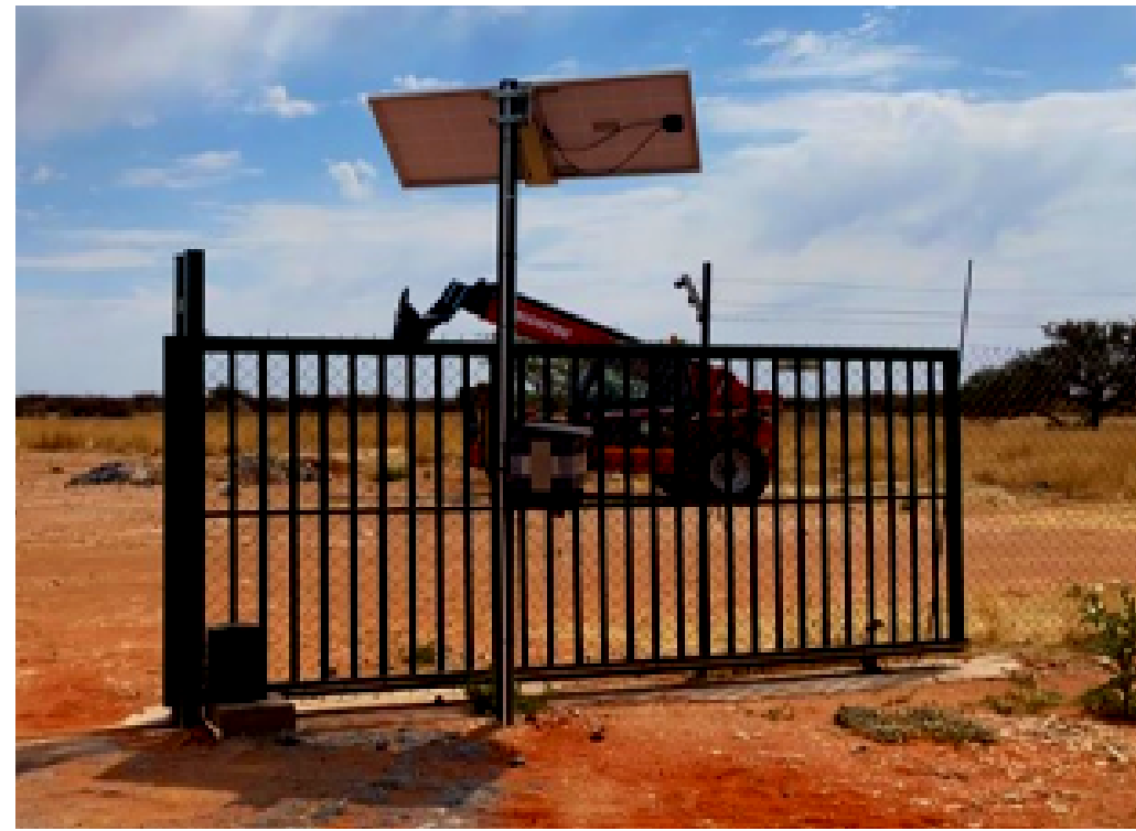
Solar Powered Gate
